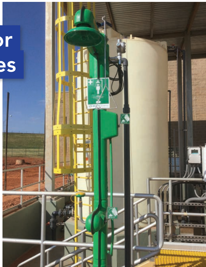
Emergency equipment must be located on the same level and within an unobstructed, 10-second walk from a potential hazard (roughly 55 feet). Image courtesy of Haws Corporation.
