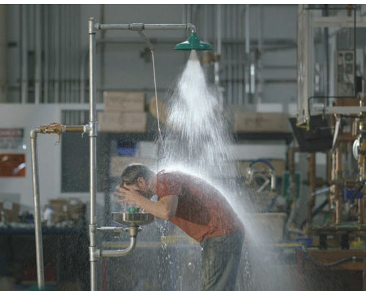
Tepid water makes it more likely that a victim will perform the required 15-minute drench or irrigation cycle. Image of facewash/shower combo is courtesy of Haws Corporation.
